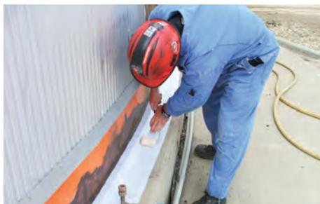
EZ WRAP, also part of InduMar's VISCOTAQ® line of products, is a unique product to seal tank chimes, roofing, air conditioning inlets and outlets. It is strengthened by a fiber mesh and having a white polyester nonwoven fiber top layer that allows for the immediate painting.
