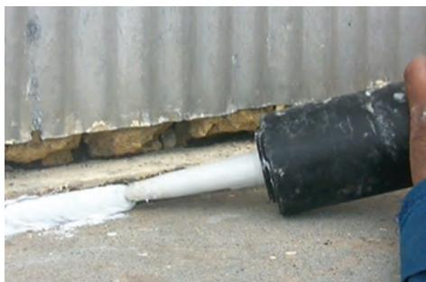
VISCOSEALANT, part of the VISCOTAQ® line of products, is a non-hardening, viscoelastic (caulk-like) compound for waterproofing and corrosion prevention. It provides a seal ring for tank chime corrosion prevention.
