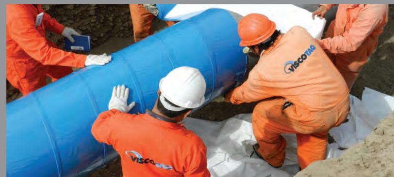
VISCOTAQ® products excel as anti-corrosive sealants because they are a synthetic viscous elastic solid. Their unique chemistry allows them to provide excellent adhesion based on van der Waals bonding principles, while being a solid with permanent wetting characteristics and eliminating disbondment.
